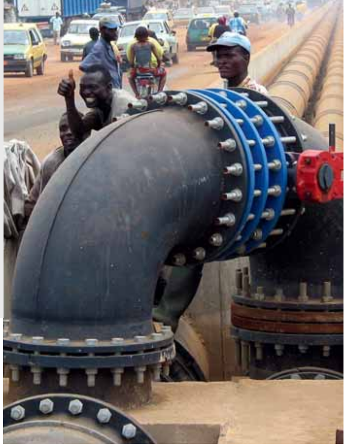
▶ Installing new water pipes in Benin
