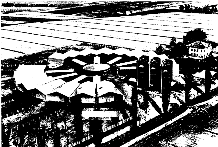
Fig. 2 — Harvestore farm in Italy. Six bunkers with rotary milking pen, screw-type fodder conveyors and open pen-barns arranged in a circle for about 1,000 animals.
