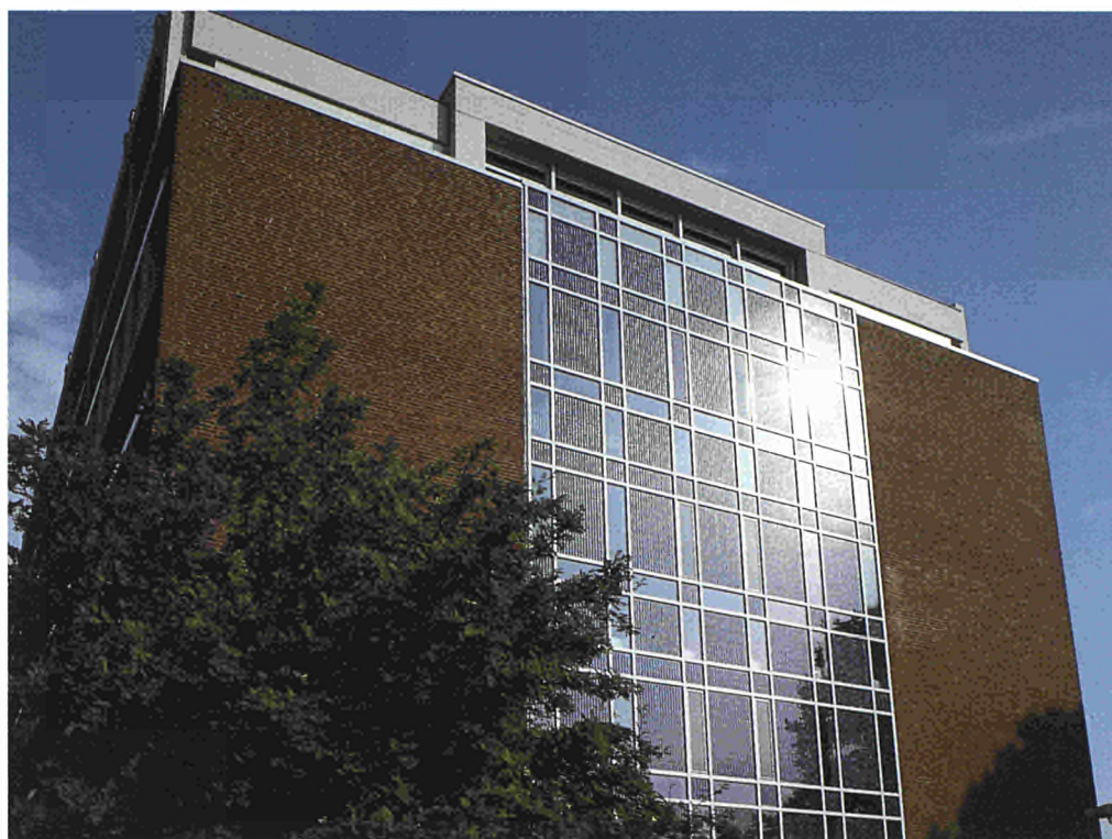
Solar façade belonging to the Aachen city authorities — an example of the use of renewable energy sources.
