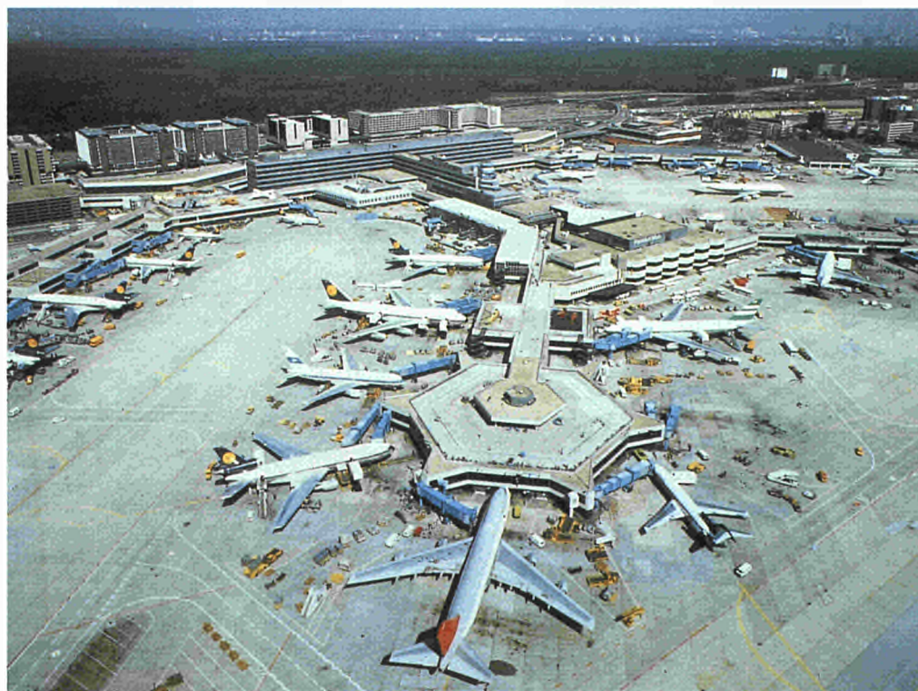
Frankfurt airport is a major hub of international air traffic and is used by 27 million passengers annually. It also provides more than 50 000 jobs.
