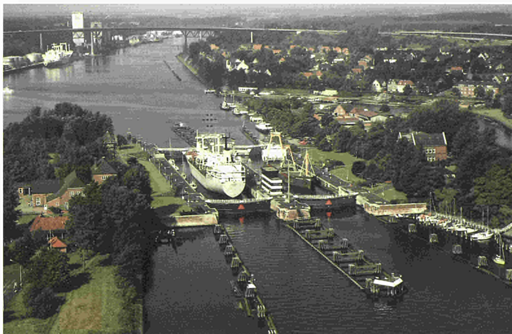
One of the two locks on the canal linking the North Sea and the Baltic Sea at Kiel-Holten; this canal is one of the busiest man-made waterways in the world (47 000 boats in 1989).
