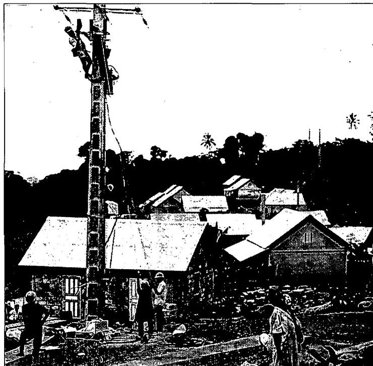
Mayotte : medium-tension rural electrification project in the village of Vahibe, financed from the 6th EDF. (Photo CEC Delegation, Mauritius)
