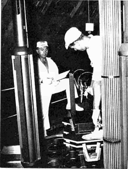
Mounting the control rods ▲
