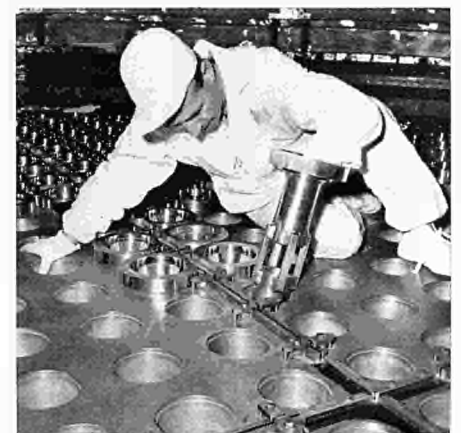
Reactor building—putting fittings into position on the reactor core support floor
