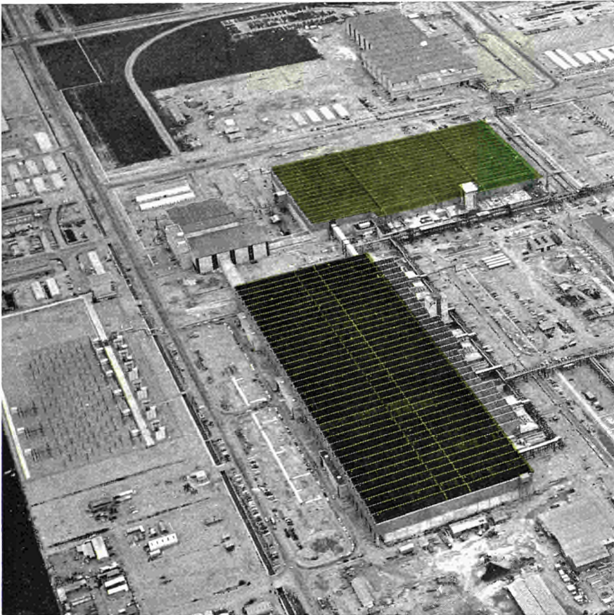
Uranium isotope separation plant at Pierrelatte. In the foreground, the low-enrichment plant; behind it the medium-enrichment plant.
