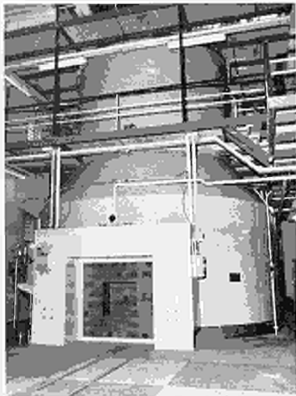
Concrete protection shield and thermal column containing the graphite of the ITAL reactor
