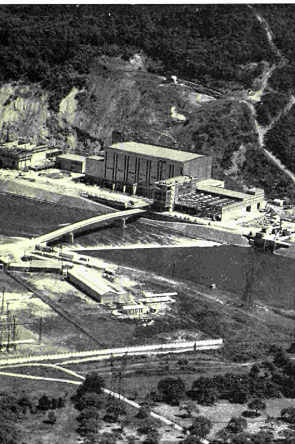
Site of the Franco-Belgian nuclear power plant in the Ardennes, at Chooz (France). The reactor and its cooling circuits are installed in two caves hollowed out of the hillside. The Franco-Belgian SENA (Société d'Énergie Nucléaire Franco-Belge des Ardennes) received joint enterprise status on 9 September 1961.
