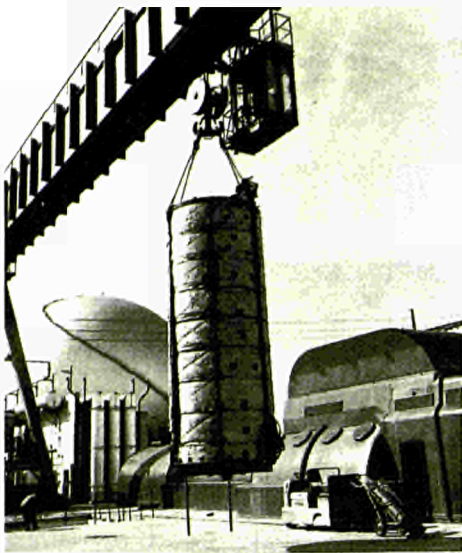
Fig. 7: Cylindrical mock-up for large-scale testing of heat insulation materials in the "Megabidon" at Chinon (France). The "Megabidon" is housed in the cavity at the bottom left of the photograph. In the background, the Chinon 1 nuclear power plant (EDF 1).
