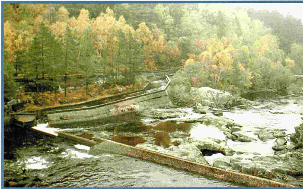
Combined infra-sound and electric fields guide salmon around a Scottish hydroelectric dam via a fish ladder (background).
