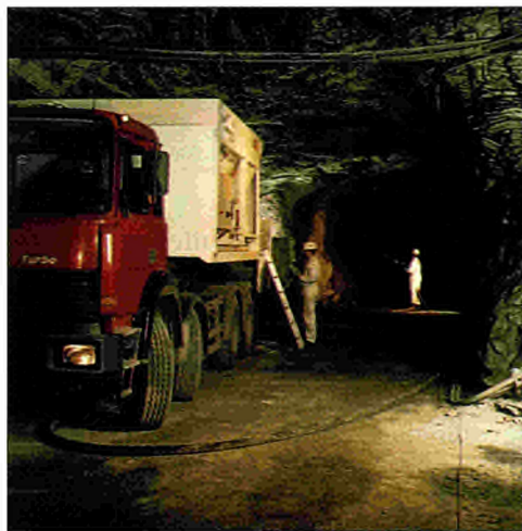
A new technology for spraying concrete onto rock when building tunnels considerably reduces the pollution of water resources and the harmfulness of working conditions.
