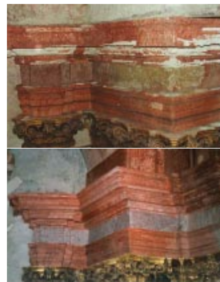
Dukes Chapel in Krzeszow before and after restoration work. Telč: the ARCHHIP centre of excellence has research units in this World Heritage City and in Prague.
