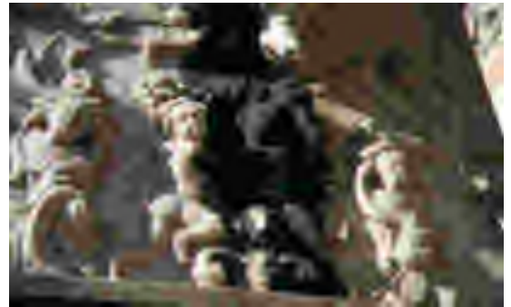
Milan Duomo: twin cherubs, one of which shows a very clearly defined area of black crust.
