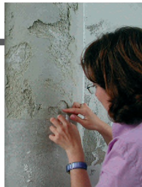
As well as its decorative function, plaster protects masonry against humidity.
