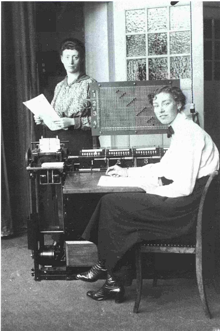
Tabulating machine, still without writing mechanism: results had to be noted manually on long lists... 1918.
