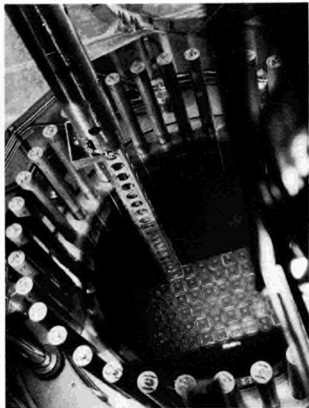
Preparations for criticality: insertion of the fuel elements in the pressurised water reactor of Obrigheim 300 MWe nuclear power plant.
