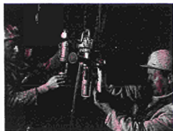
Use of tyndalloscope and konimeter for dust-measurement (see p. 77).
