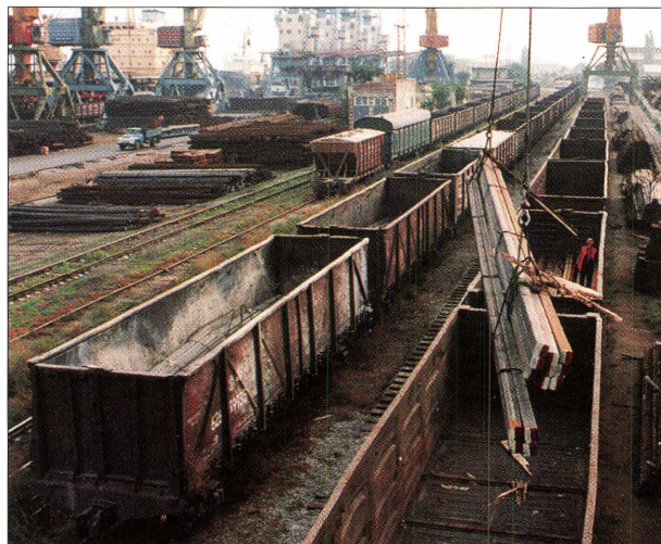
The terminal at the port of Odessa is working at half capacity due to the poor state of facilities. A Tacis project is preparing detailed studies on a centralised computer cargo handling system and training managers and technicians
