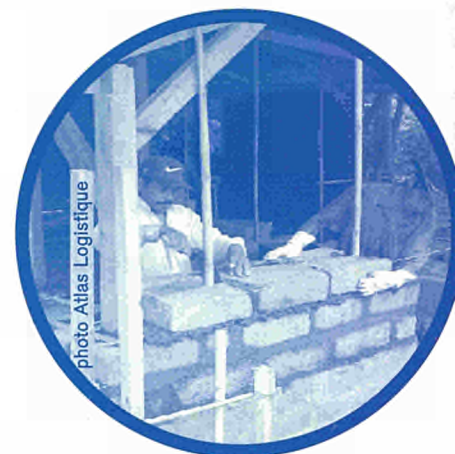
House reconstruction in Salvador - ECHO project -
