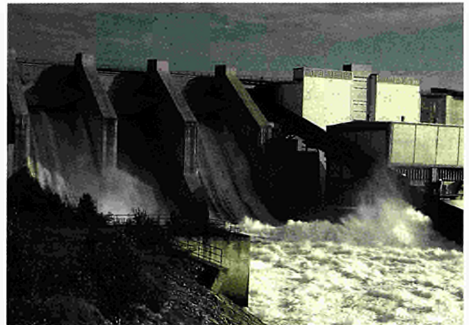
Hydro-electric power station in northern Sweden
