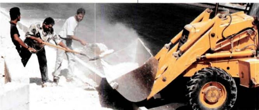
Rehabilitating the road network in Gaza
