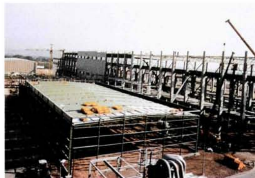
Construction of a corrugated cardboard production plant near Zaragoza
