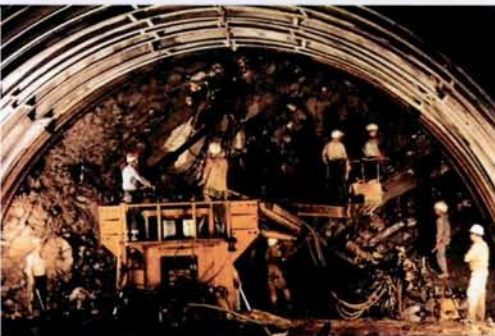
Building the Athens metro
