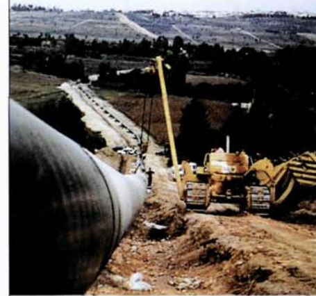
Extending the natural gas network
