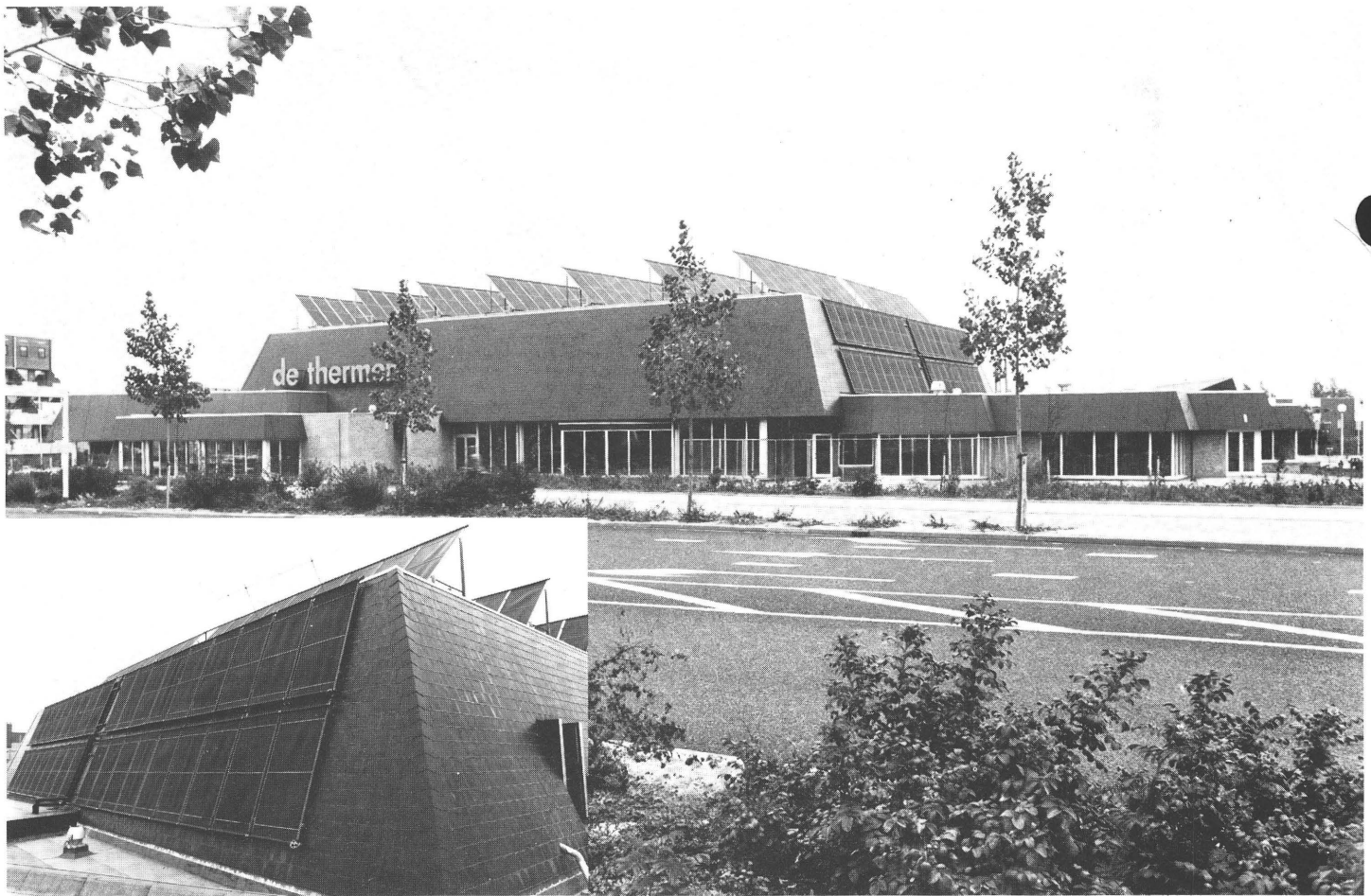
'De Thermes' solar heated swimming pool, Alphen aan den Rijn, The Netherlands (SE/P/4/81)
