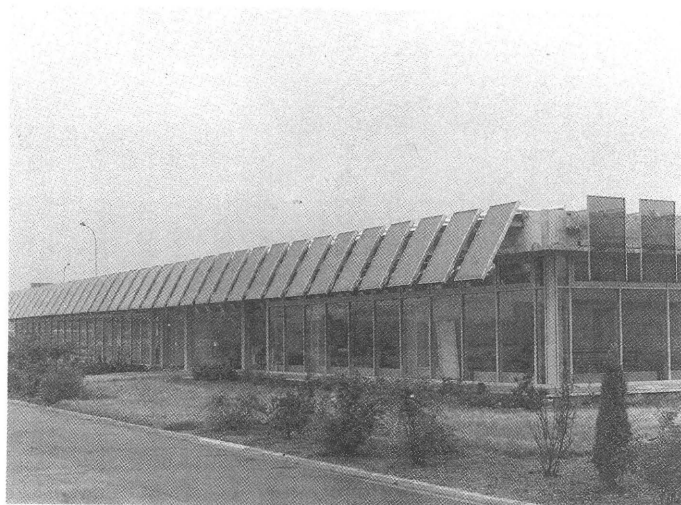
Facade mounted collectors in Fleurus, Belgium (SE/131/79)
