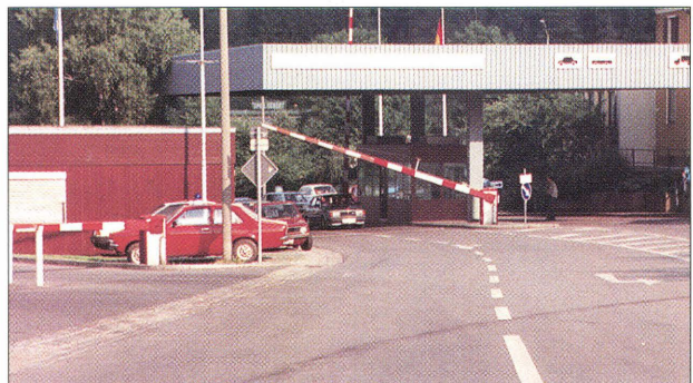
The Phare cross-border initiative strengthens regional links between Phare partners and their EU neighbours. Upgrading of roads and customs facilities are two key responsibilities.
