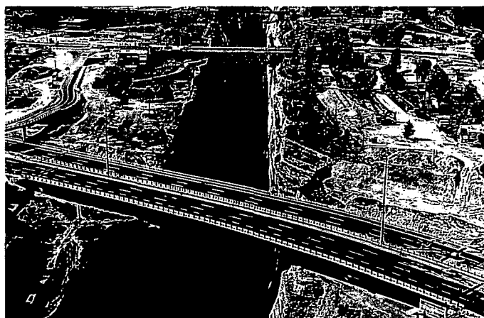
PATHE trunk road: bridge over Corinth Canal
