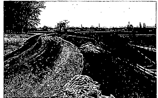
Strengthening of dykes in Gelderland
