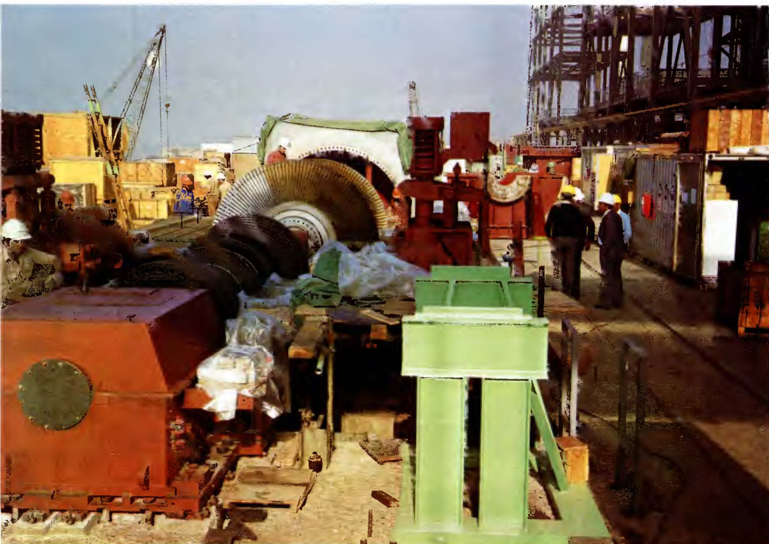
Fitting out the Ait Chouarit-Amougeez hydroelectric complex in Morocco (Operation No 261).
