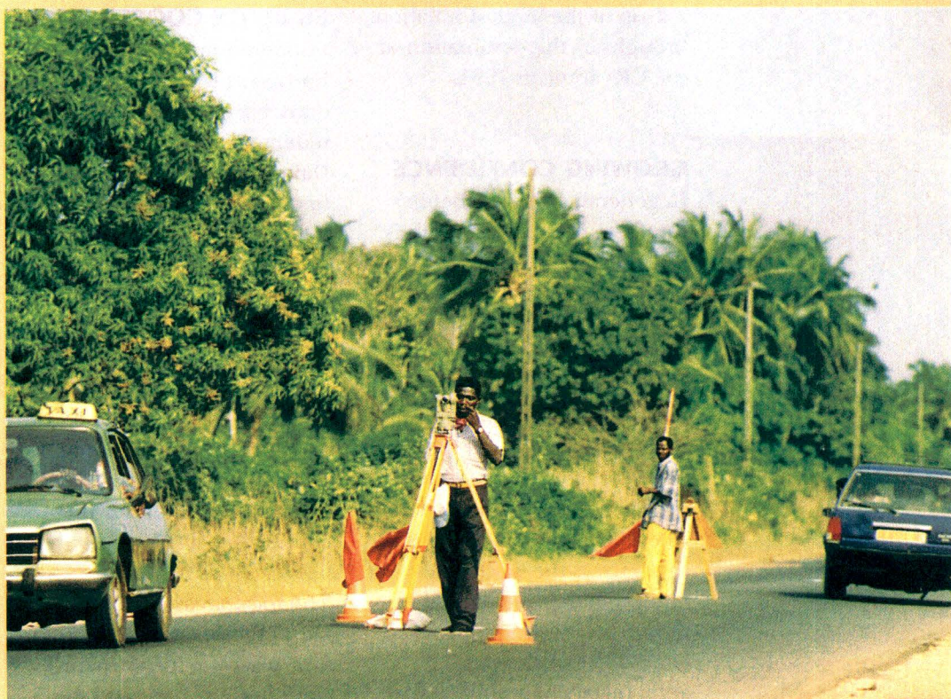
Benin. Work underway on the Cotonou-Lomé road.
